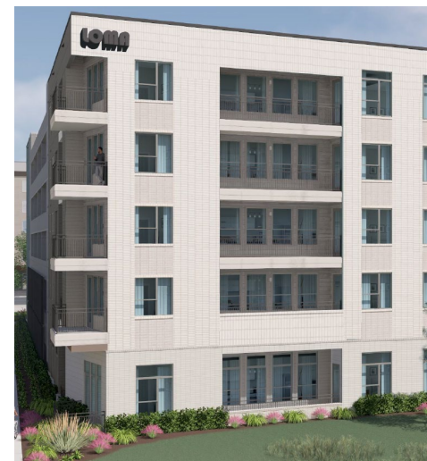
Oakhouse Phase II (Loma) – Dallas, TX
